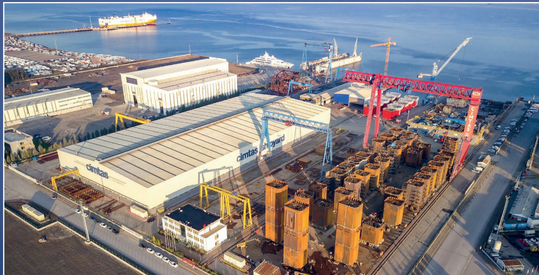
TOWER BLOCK TRIAL ASSEMBLY
