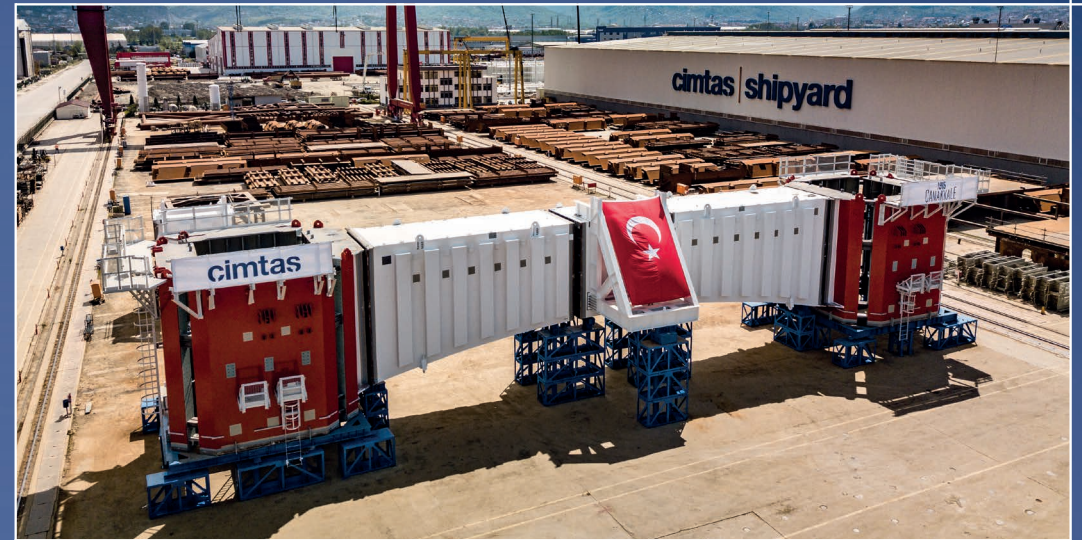
TOWER CROSS BEAM TRIAL ASSEMBLY
