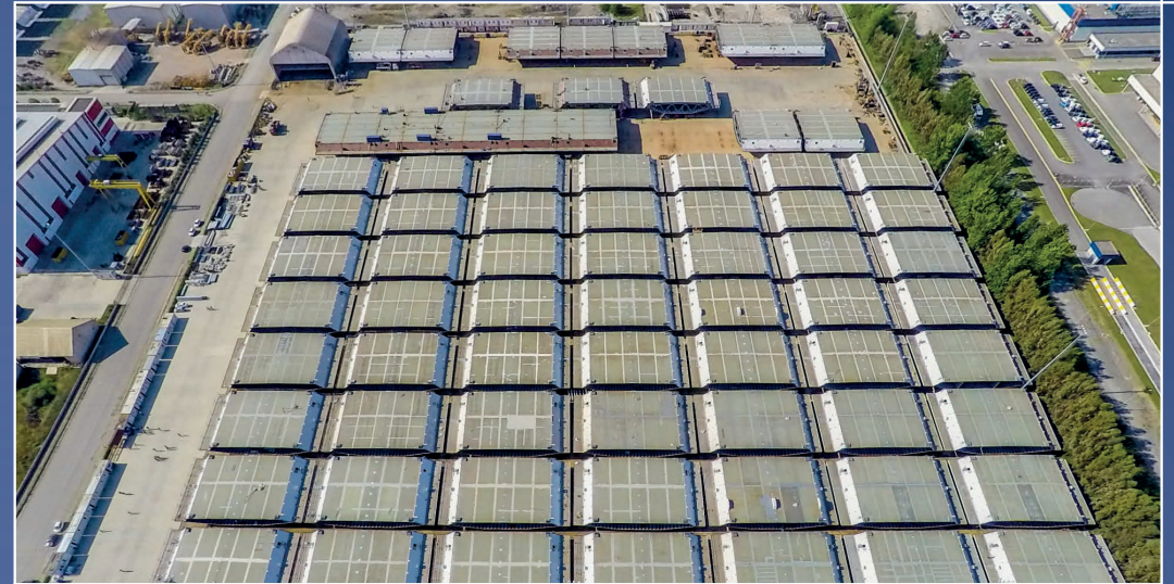
GIRDER BLOCK TRIAL ASSEMBLY & STORAGE
