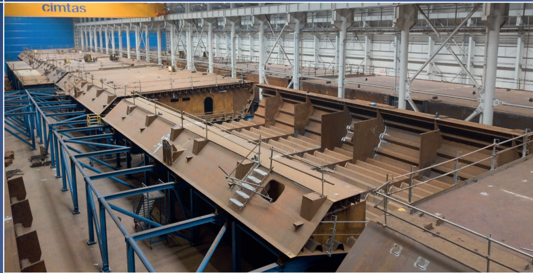
GIRDER BLOCK FORMATION
