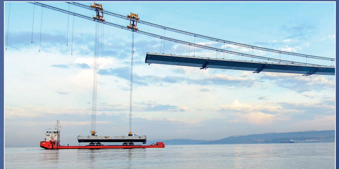
GIRDER BLOCK TRANSPORTATION
