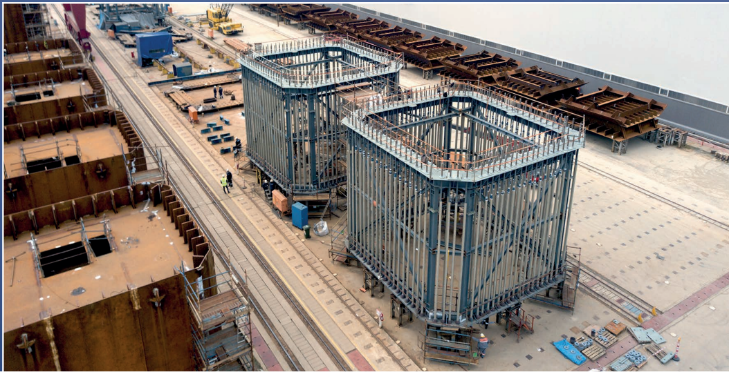
ANCHOR FRAME FABRICATION
