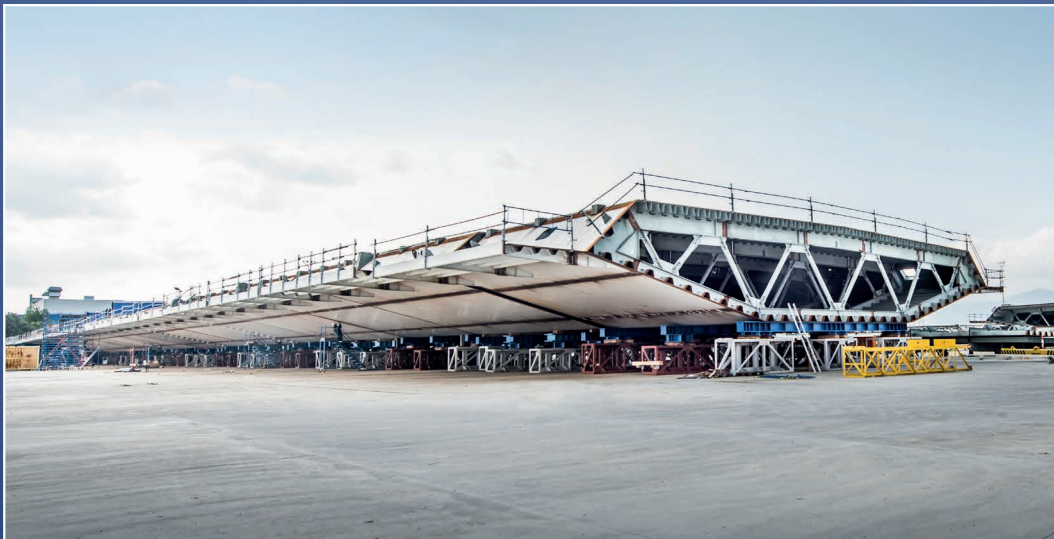
GIRDER BLOCK TRIAL ASSEMBLY
