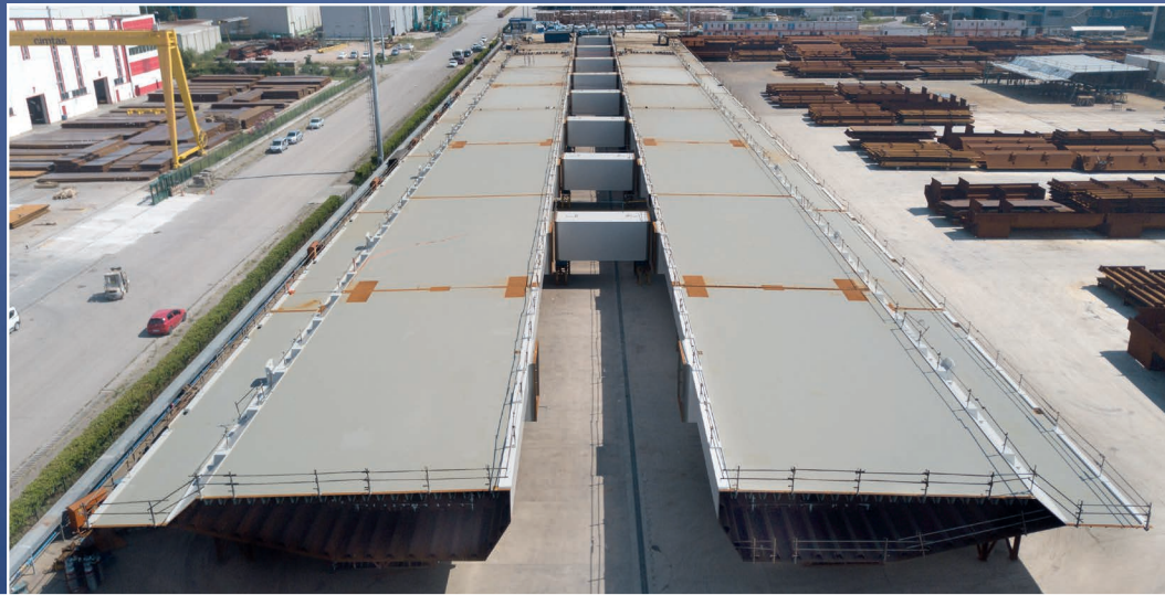
GIRDER BLOCK TRIAL ASSEMBLY
